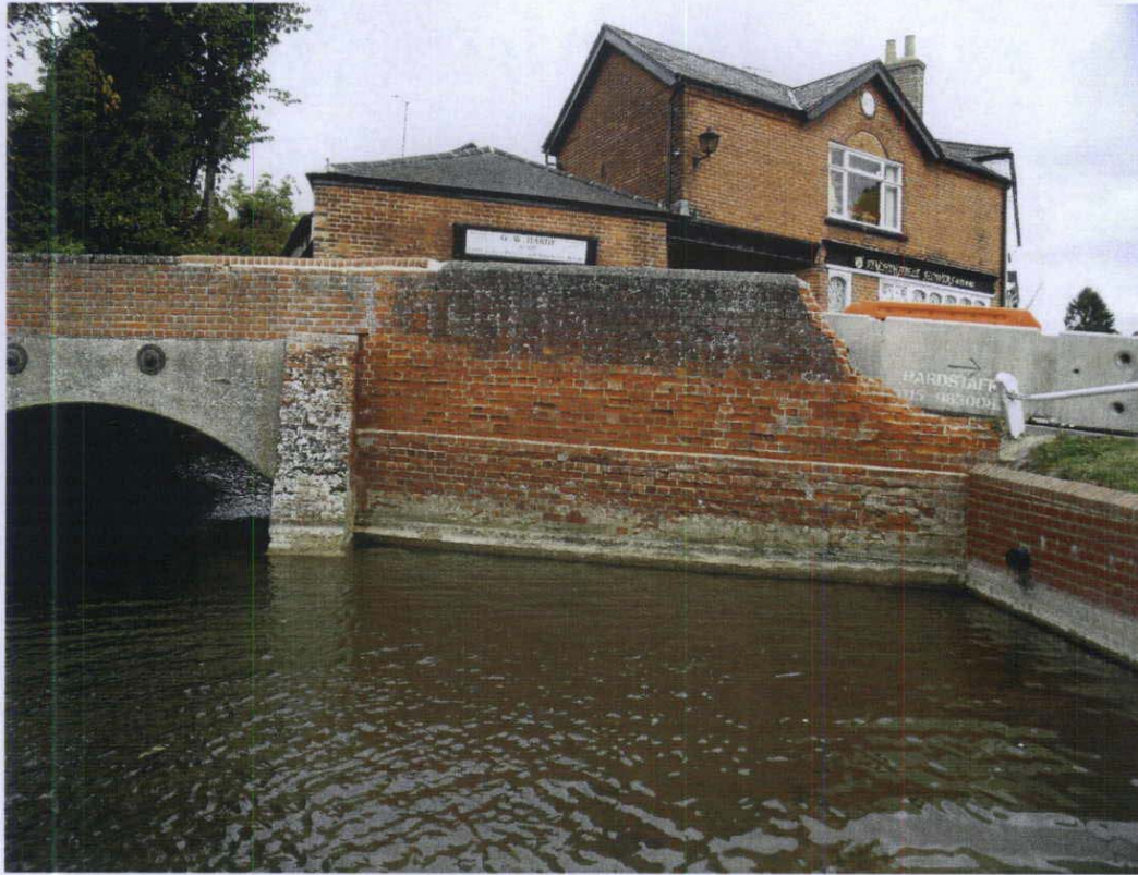
Photo No. 9 – Southeast Wingwall & Parapet
