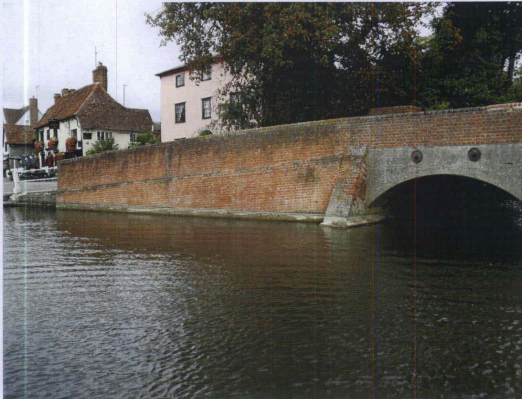
Photo No. 8 – Southwest Wingwall & Parapet
