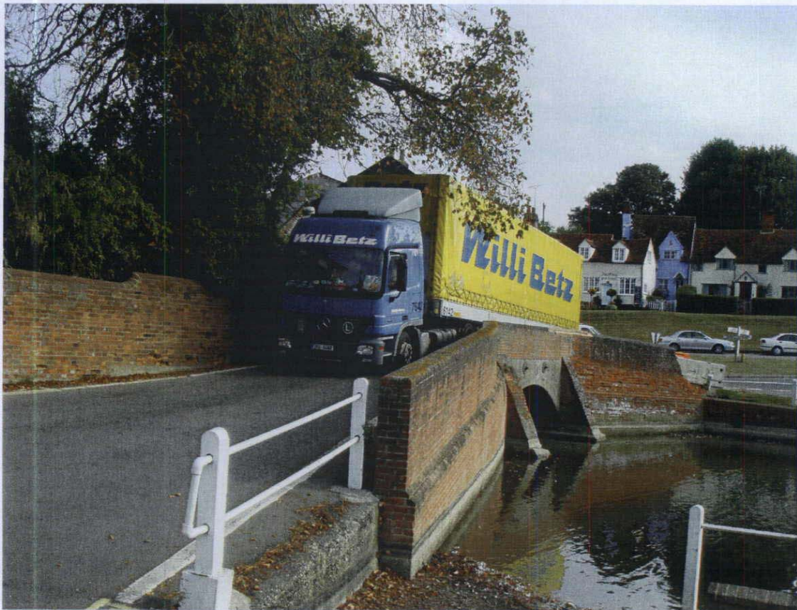
Photo No. 2 - View of HGV crossing structure
