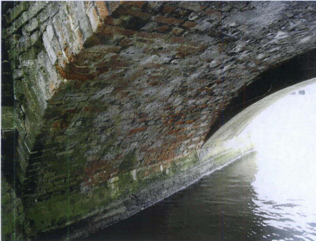
Photo No. 6 - View of masonry arch springing (east)
