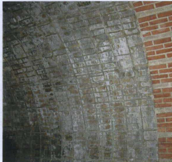
Figure 2 – Masonry Arch Repair System (Completed Installation)
