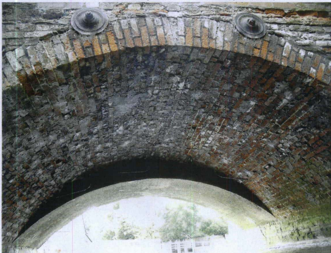
Photo No. 4 - View of the original brick arch from North (downstream)
