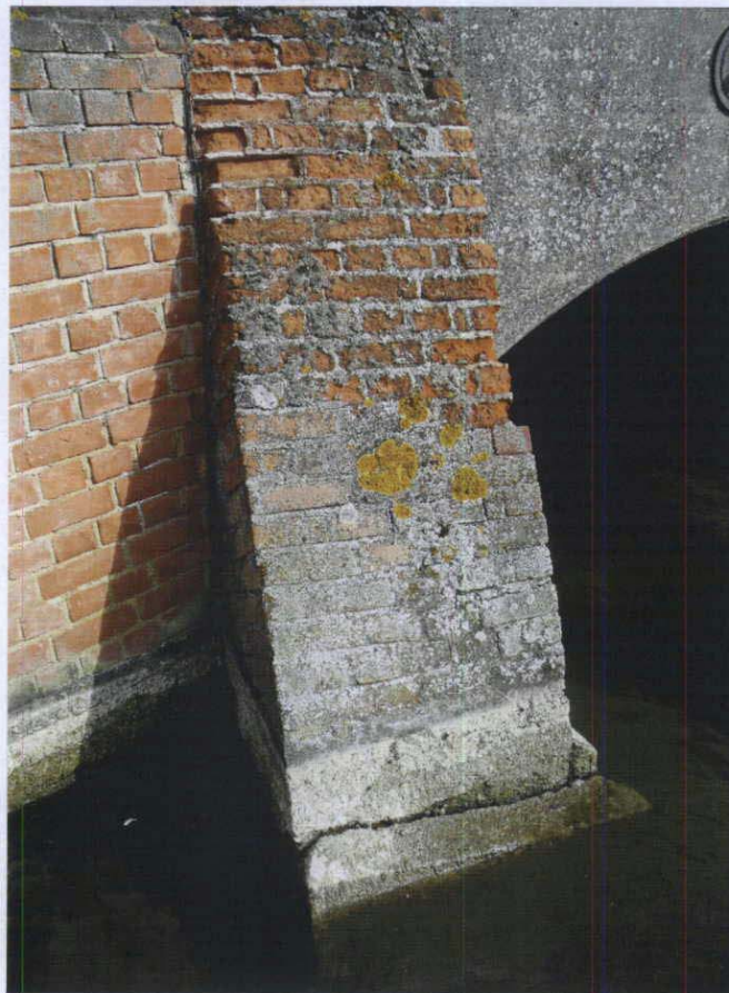
Photo No. 10 - View of Southwest buttress
