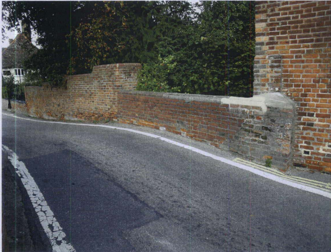
Photo No. 7 – North Parapet
