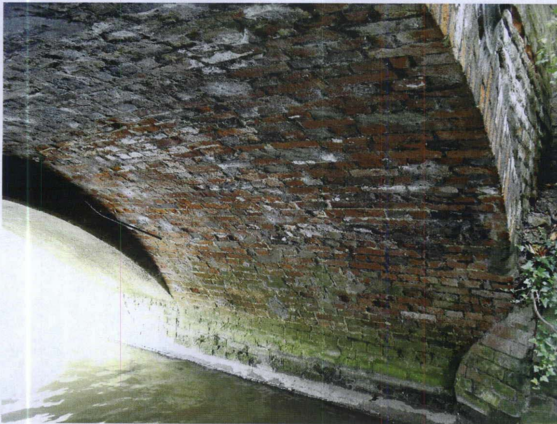
Photo No. 5 - View of masonry arch springing (west)
