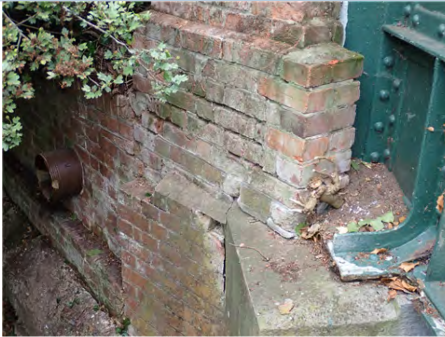
North West Pilaster (south face) Ivy stump adjacent pilaster.
