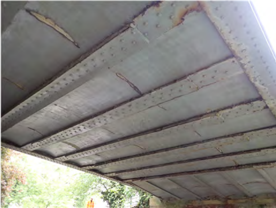
North West Corner Deck Soffit (looking SE)
