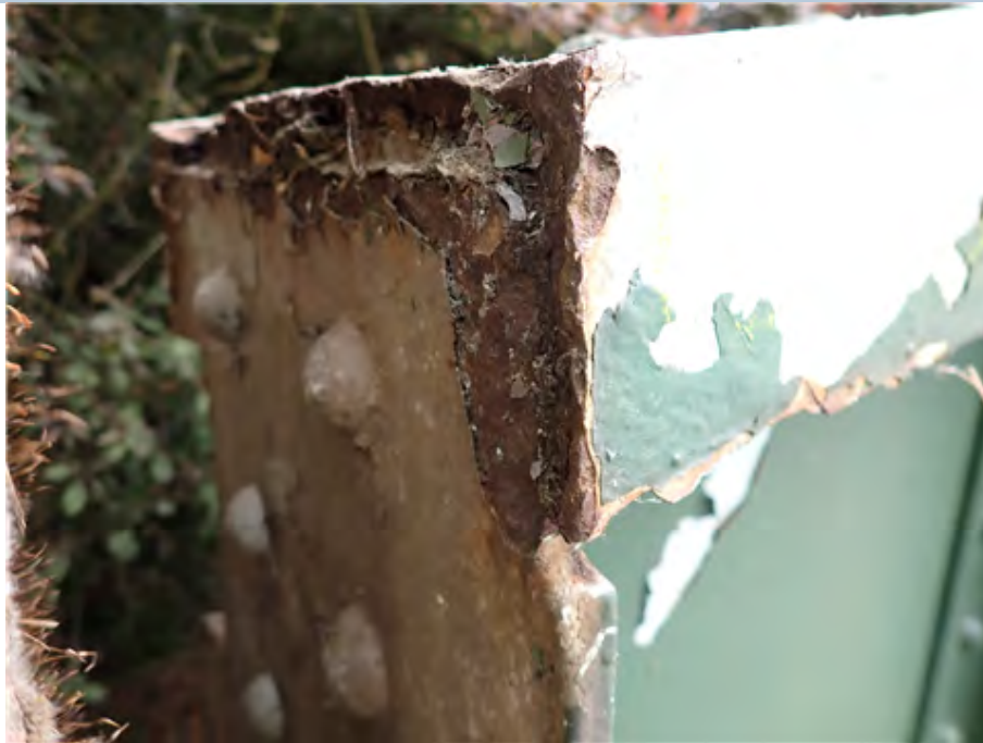
East Edge Girder Top Flange (north side)
