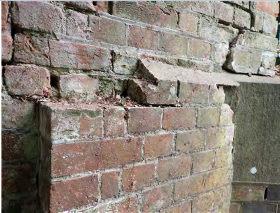
North West Pilaster (west face lower section)
