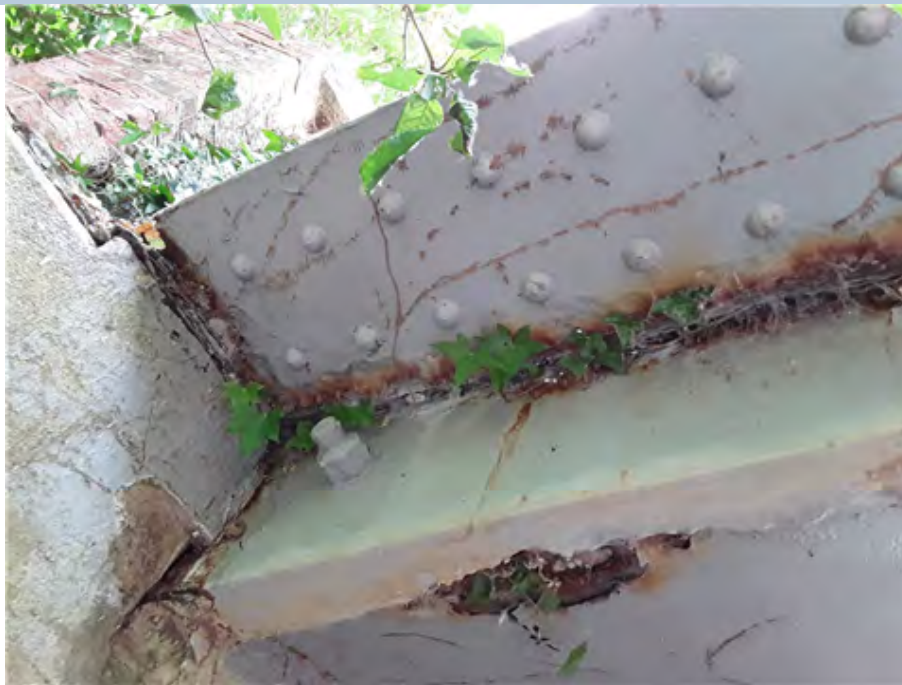
East Edge Girder Bottom Flange (south side)
