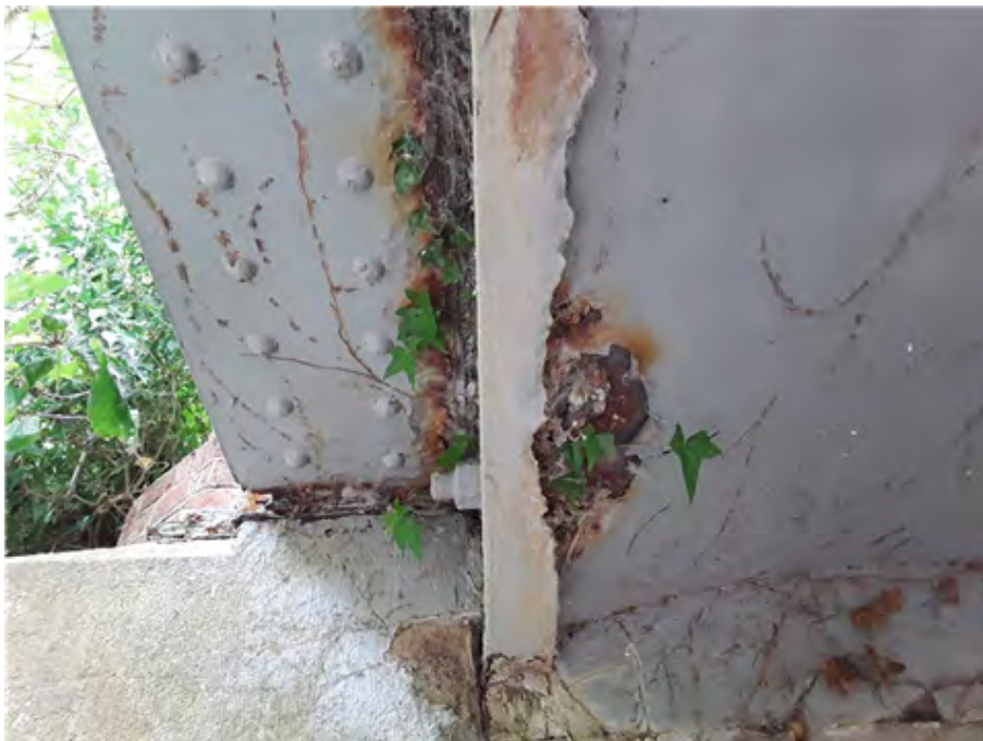
East Jack Arch at South End.
