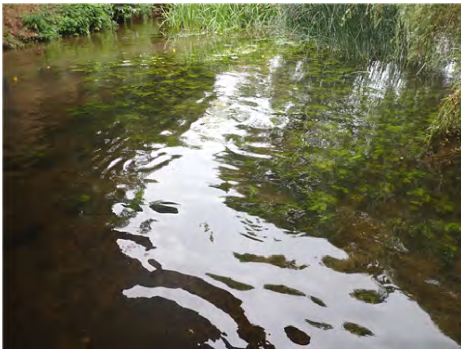
West River Bed (midspan) Minor scour, slightly deeper area of river bed.
