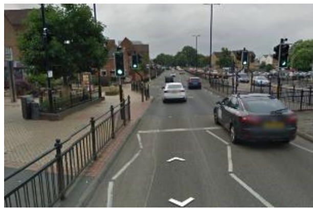
Image 6 – South-eastbound carriageway crossing
