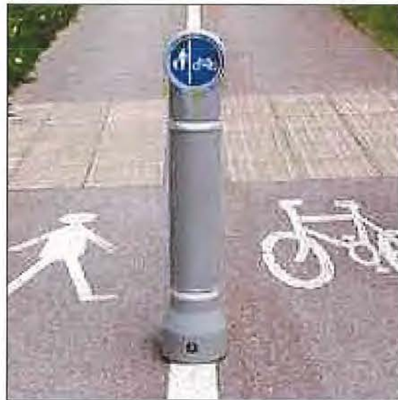
Proposed Bollard B - to be black in colour (with segregated Cycleway/Footway roundel on both sides)
