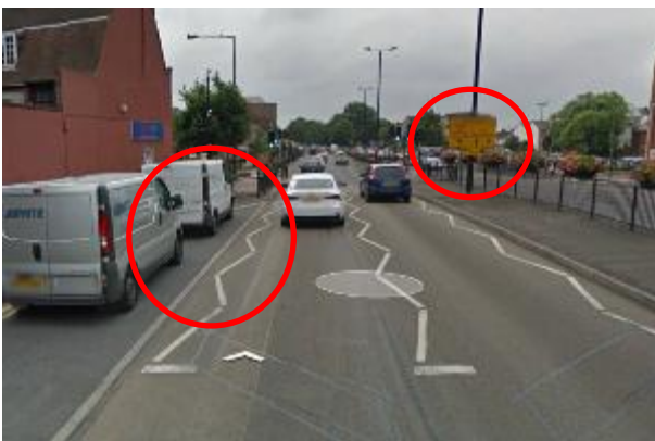
Image 5 – South-eastbound approach (parked vehicles masking pedestrians approaching the crossing and temporary diversion route sign on central reserve)
