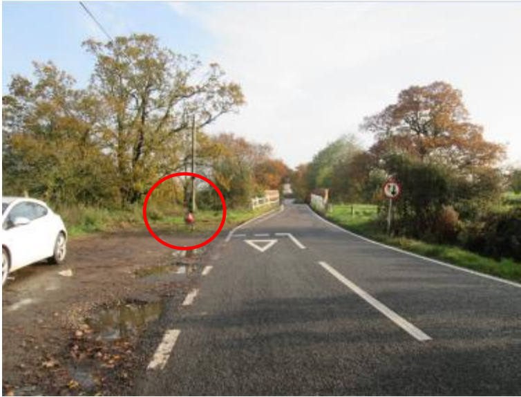
Image 3 – Southbound approach to bridge (road narrows from nearside only and damaged sign)
