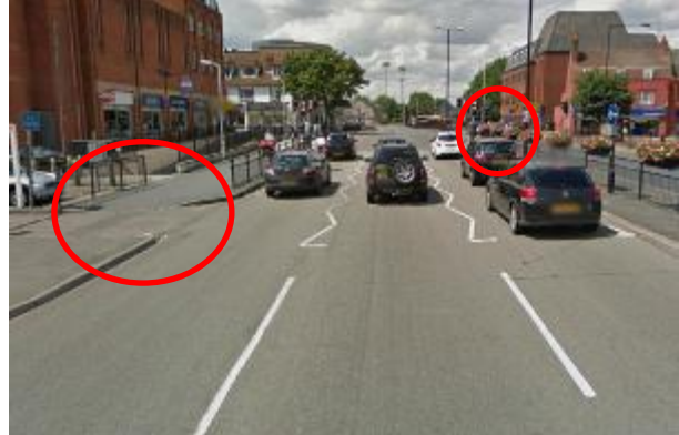
Image 2 – North-westbound approach (exit from car park on nearside and planters mounted to guardrail on offside)
