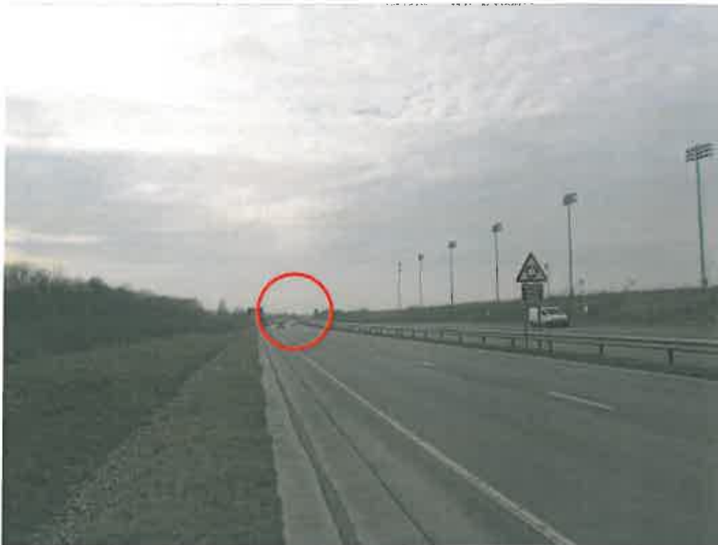
Photograph 1: A131 southbound approach to the Moulsham Hall Lane Roundabout, Great Leighs.
