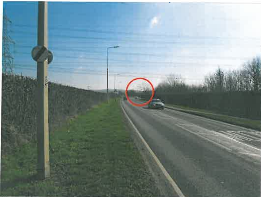
Photograph 1: View travelling eastbound on the A1060 Maldon Road towards the junction with Brick Kiln Road located on the offside.
